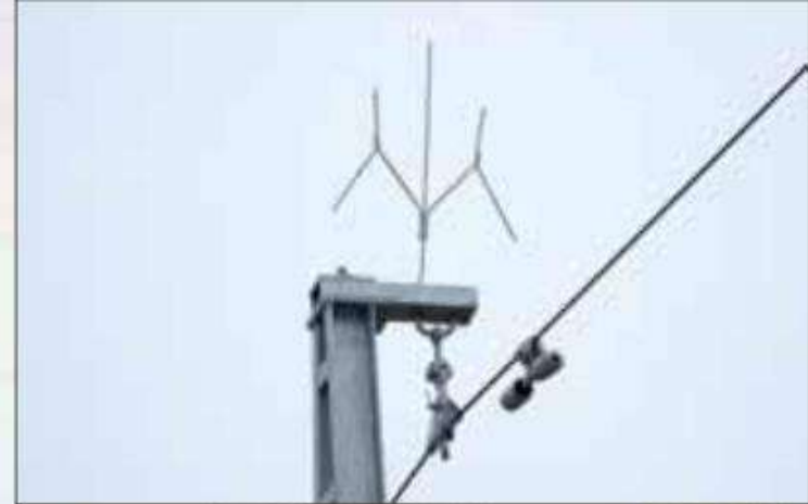
Wishbone Prevents Bird Landing on Wire
